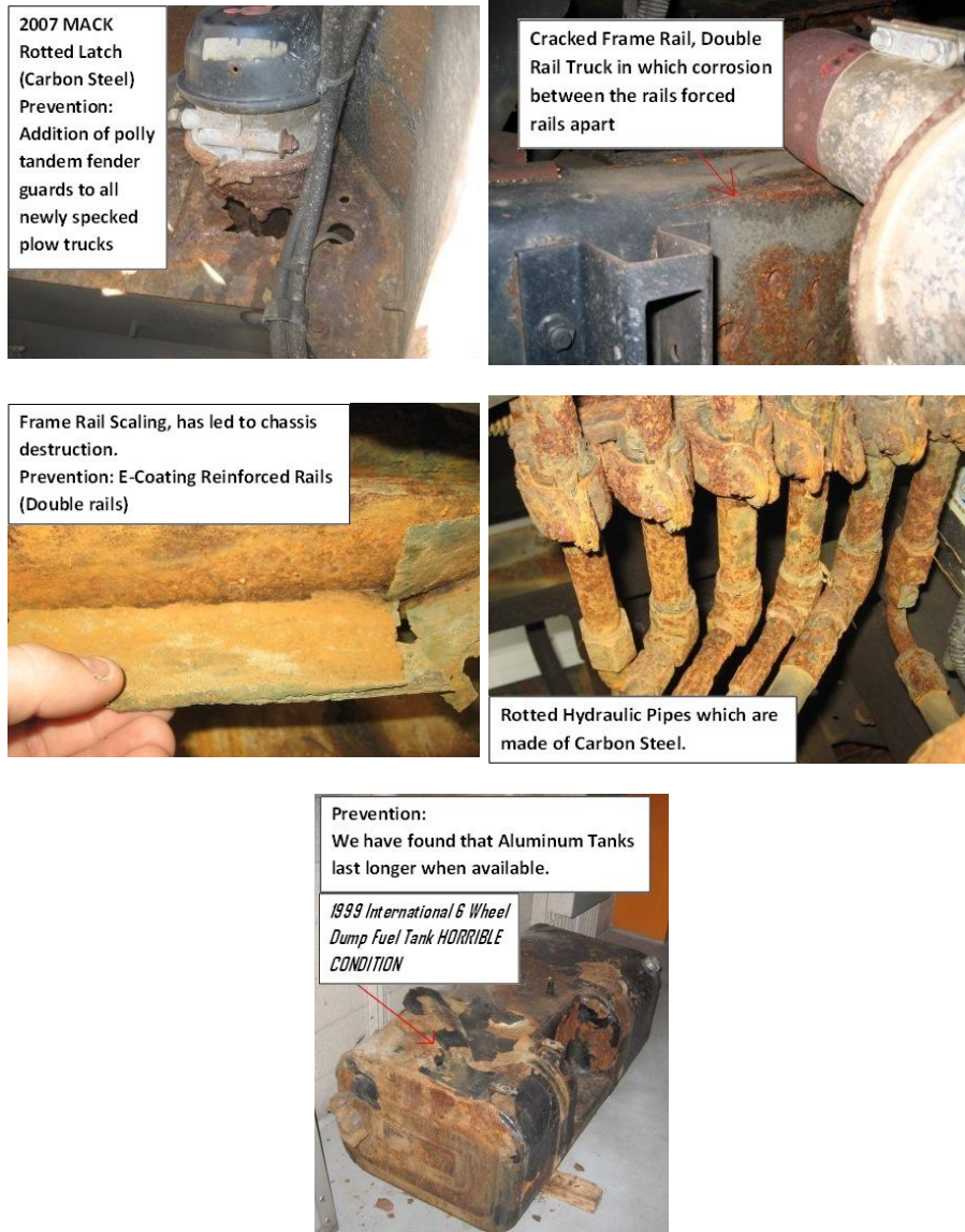
Figure 24. Images of corrosion damages on RIDOT vehicles (courtesy of RIDOT).
