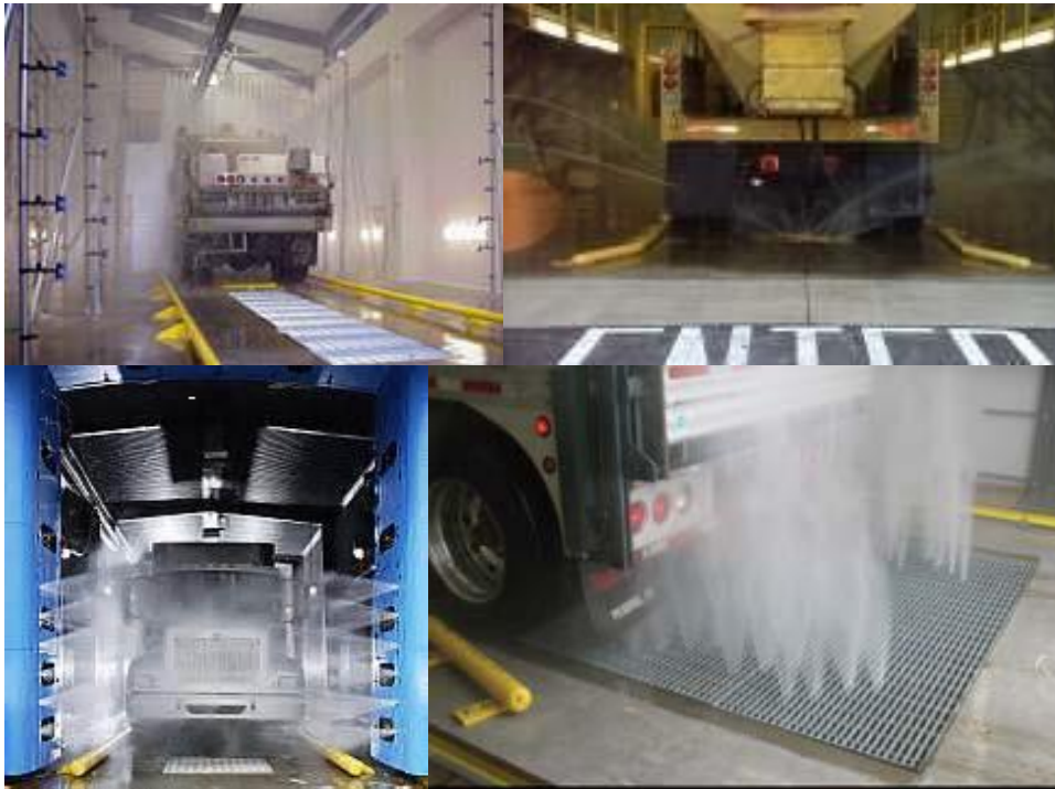
Figure 43. Automated truck washing (Clonch, 2014; Chupas, 2014).
