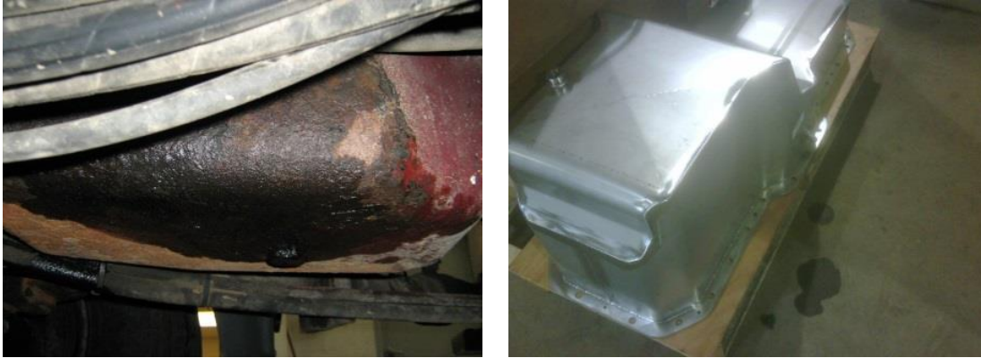
Figure 48. Corroded oil pans (left), and replaced by stainless steel (right) (Smith, 2014).
