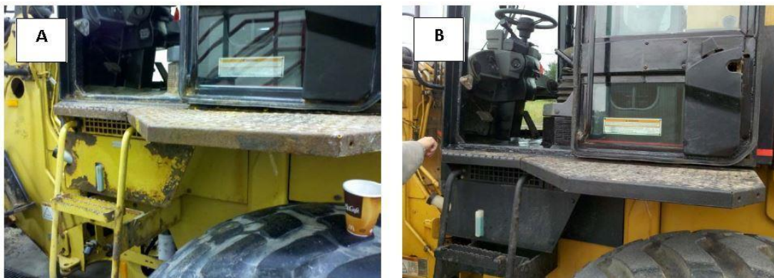
Figure 40. Corrosion damage on a winter maintenance vehicle (a), and in-field success of UV curable coating (b) (Monty et al., 2014).
