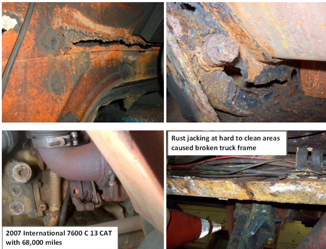
Figure 27. Images of corrosion damages on ConnDOT vehicles (Chupas, 2014).
