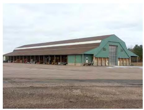
Photo#1: This facility in Washburn County, Wisconsin, houses both state and county salt supplies, with a wall in the center of the building to keep the stockpiles distinct.
