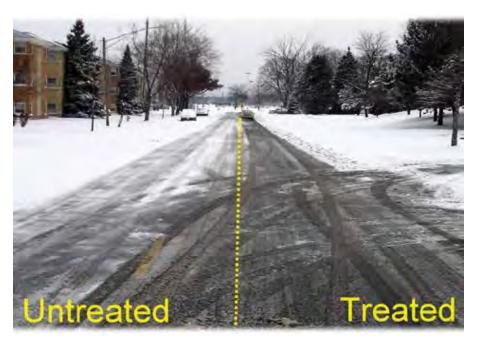
Photo#3: Anti-icing can reduce salt usage by up to 75 percent if conditions are right. The manual includes a flowchart to help determine whether anti-icing is likely to be effective.
