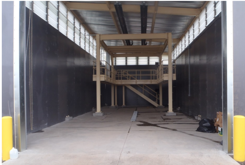
Photo 1: Vehicle wash facility completed 2015
