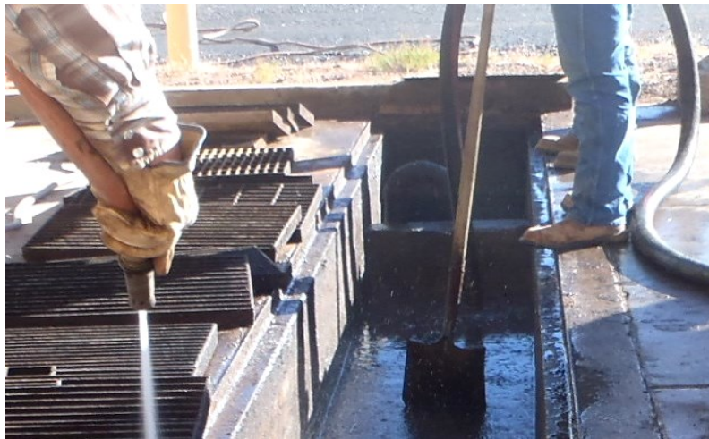
Photo 3: Trench with sediment removed
