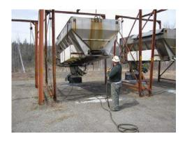
15) Whenever possible, the hopper should be completely washed after removal. **Note:** Wear all appropriate PPE.
