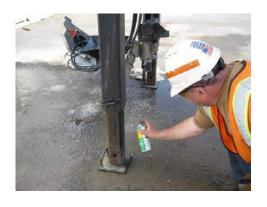
A liberal amount of graphite shall be applied to the portion of the rear legs that slide into the hopper stand frame.
