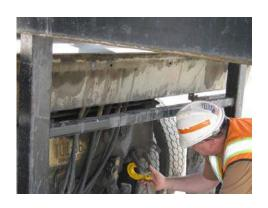
6) At this point, the spotter will indicate that he is going under the hopper to attach the limiter strap to the truck. The strap is designed to prevent the hopper from coming out of the body before the legs are down and locked. Check the strap to ensure it has been adjusted to the proper length. Note: The legs of the hopper stand device are still in the down and locked position.
