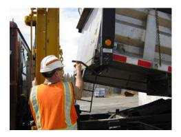
12) The spotter will then direct the operator to lower the body completely.
