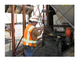
9) The spotter will then hook the chain falls located on the gantry to both sides of the rear of the hopper. Note: The spotter will remove all slack from the chains by adjusting the chain falls.
