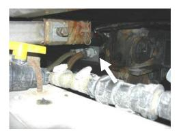
7) To complete the spinner assembly installation, connect the liquid/brine fittings
