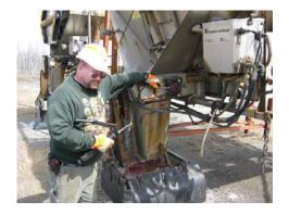
3) Before positioning the truck for the installation, check the hopper for mechanical issues and grease the hopper if necessary or scheduled.
