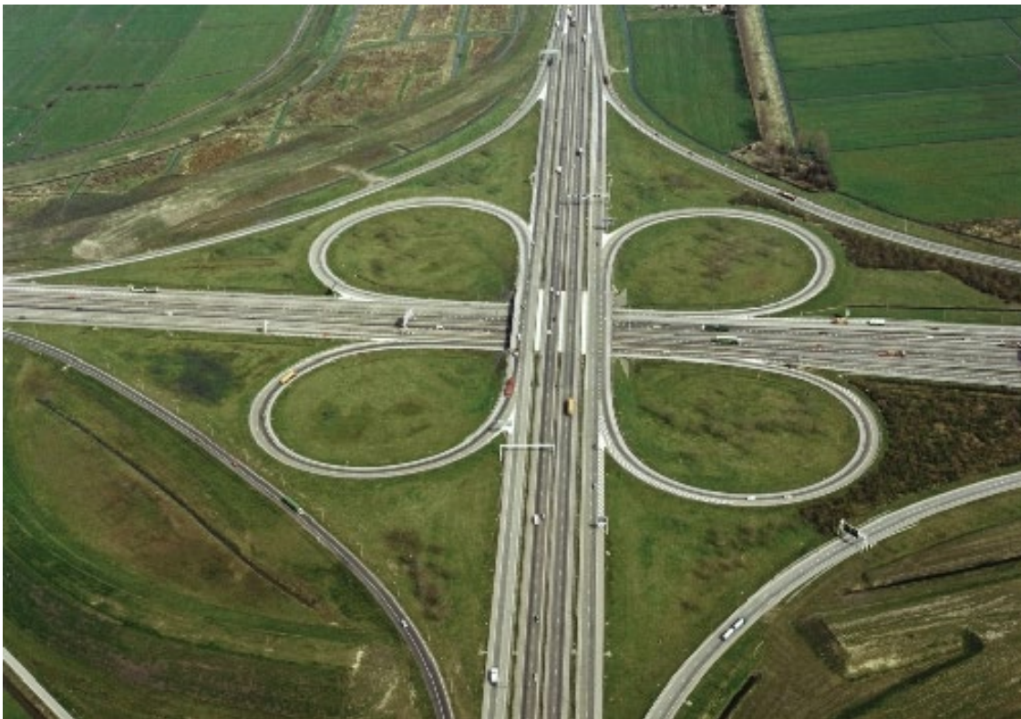
Figure 8.1: Cloverleaf interchange
