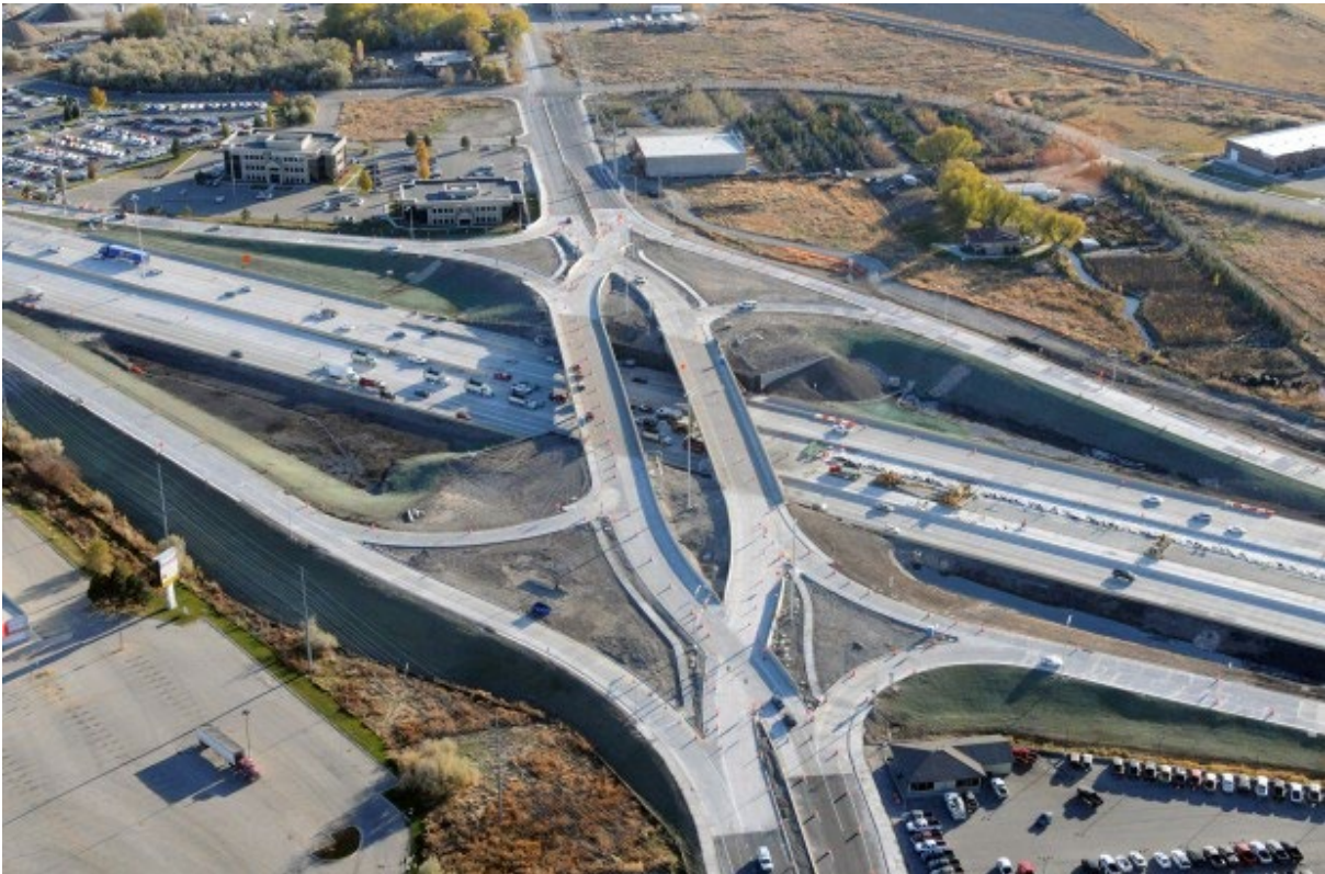
Figure 10.1: Diverging diamond interchange
