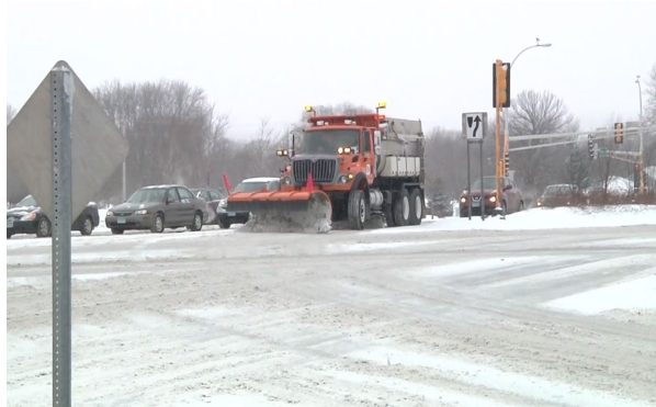
Figure 1.1: Snow plowing an intersection
