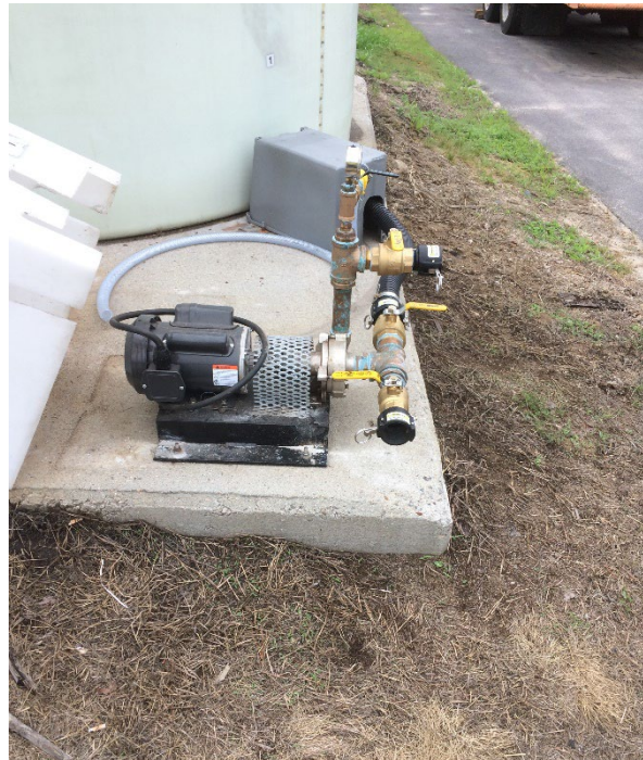
Figure 27: Pump/Motor Set Up on Metal Plate
