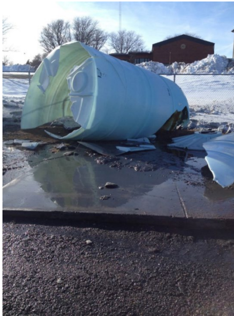
Figure 24: Poly Tank Rupture
