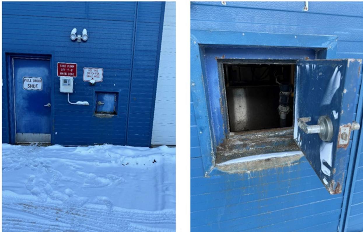
Figure 15: Brine Building Access Door
