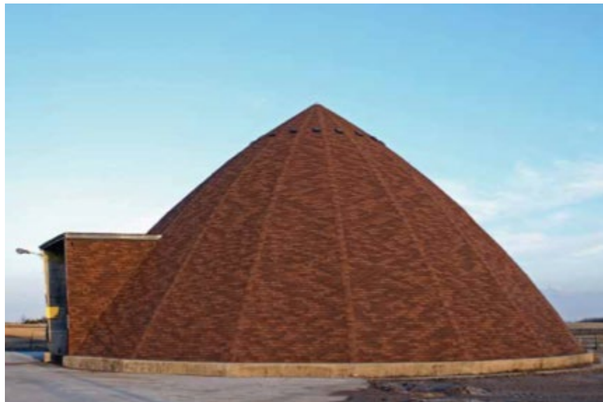
Figure 8 Conical Storage Facility
