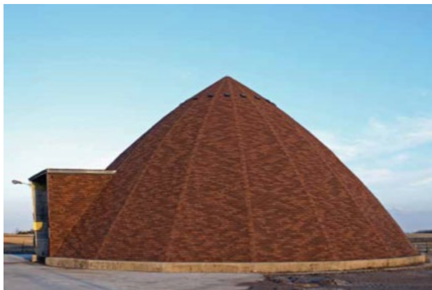
Figure 2 Salt Storage Dome
