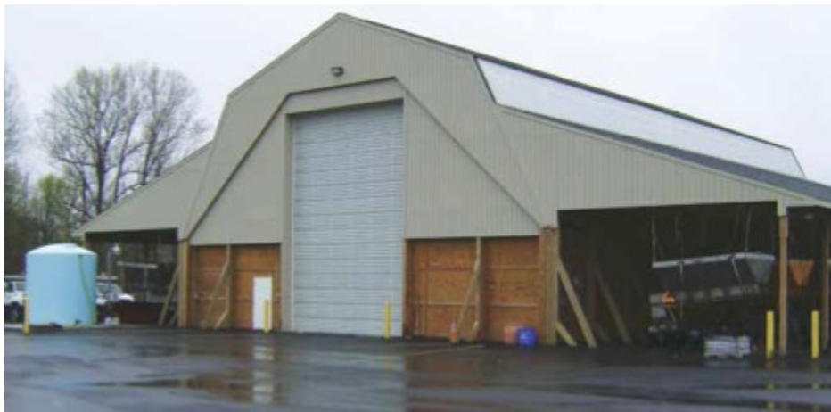
Figure 3: Rectangular Storage Facility
