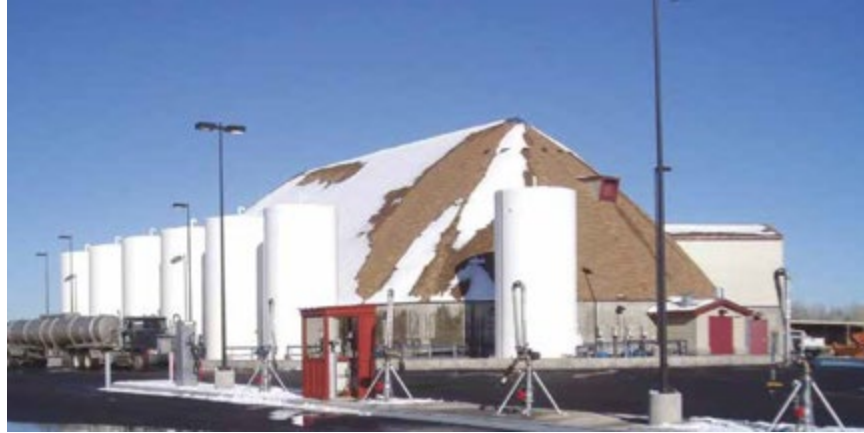
Figure 9 Elongated Conical Storage Facility
