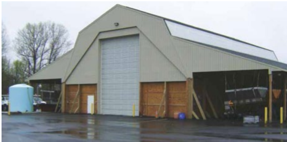
Figure 10 Rectangular Storage Facility
