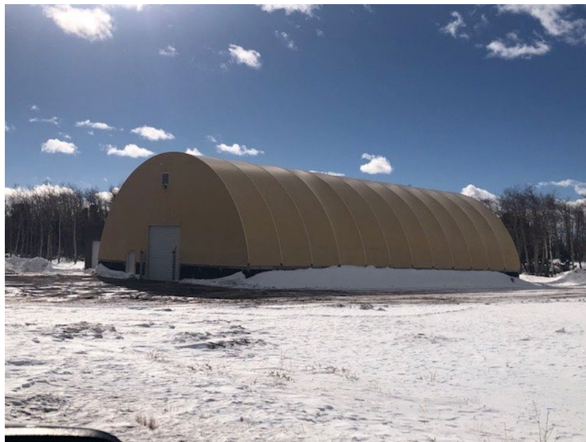
Figure 11 Fabric Covered Salt Storage Facility (courtesy of WYDOT)
