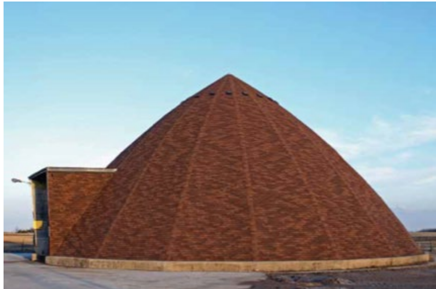
Figure 1: Conical Storage Facility
