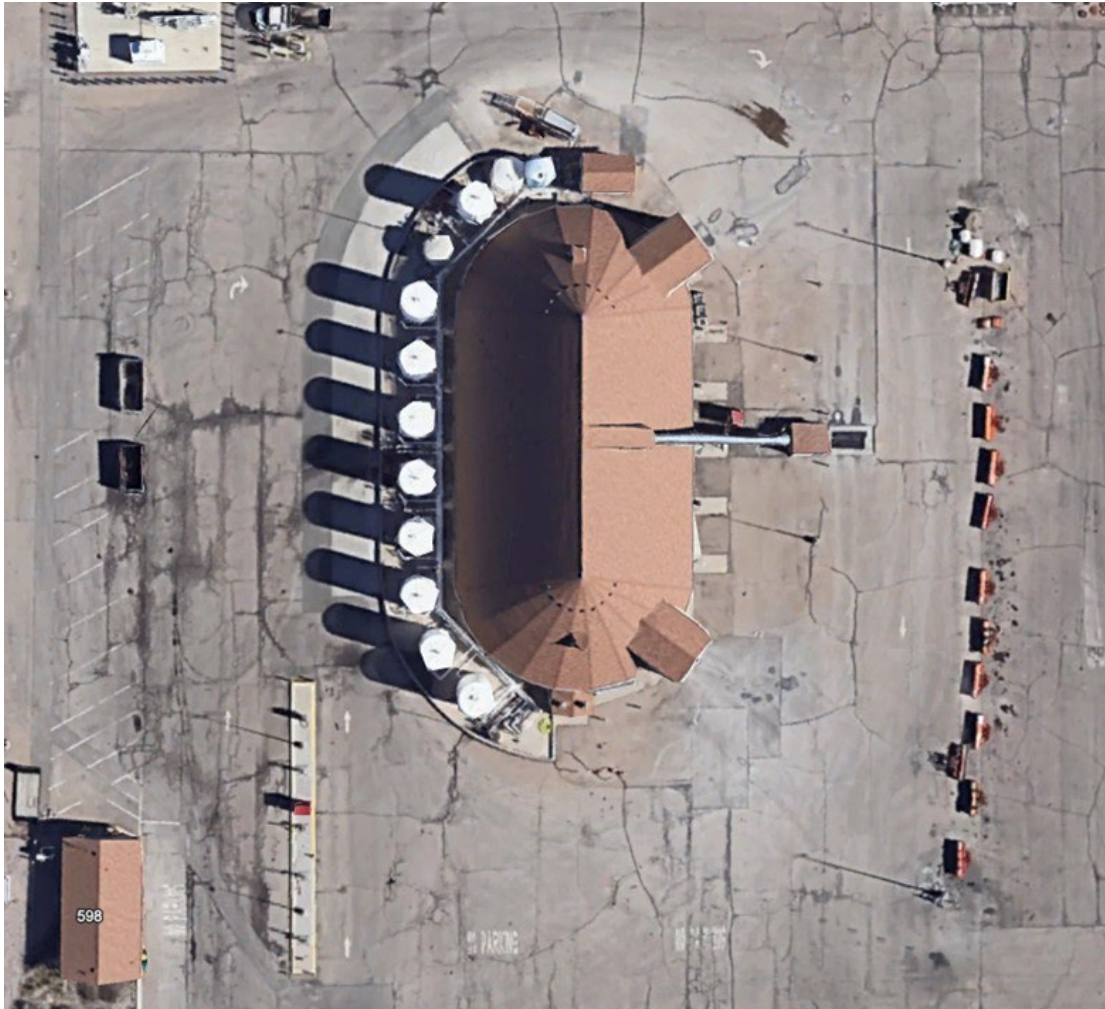
Figure 5: Salt Storage Facility showing Good Site Layout for Loading and Unloading.
