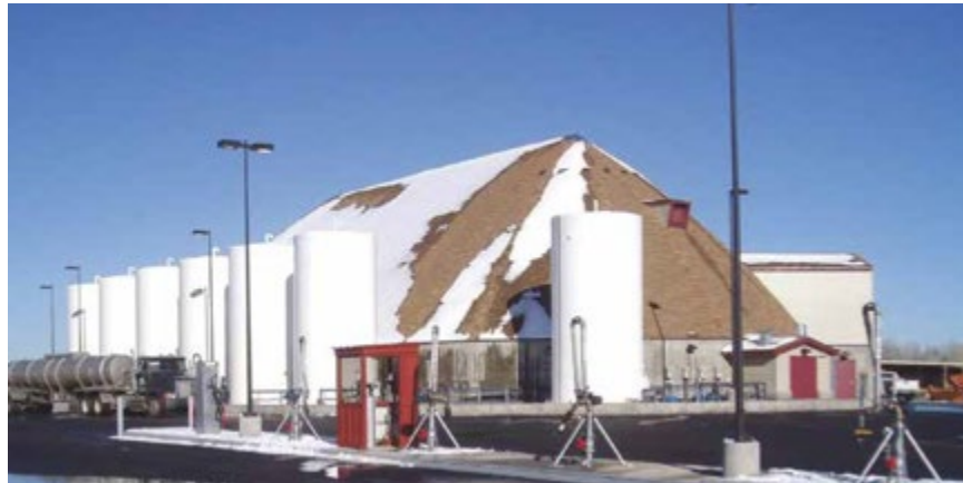
Figure 3 Elongated Salt Storage Dome
