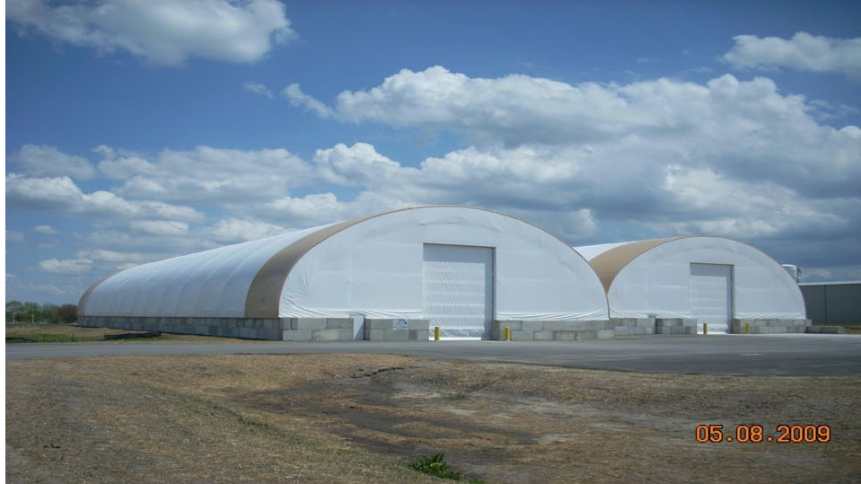
Figure 5 Fabric Covered Salt Storage Facility
