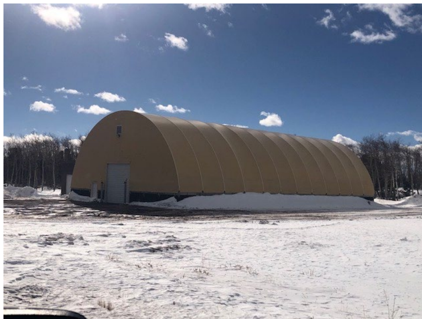
Figure 4: Fabric Covered Salt Storage Facility (courtesy of WYDOT)
