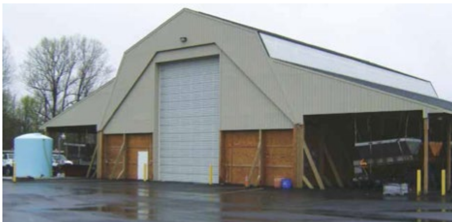
Figure 4 Salt Storage Shed (essentially rectangular)
