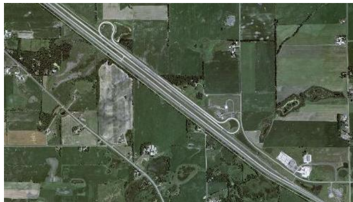
Figure 21. Aerial View of MnROAD Test Facility
