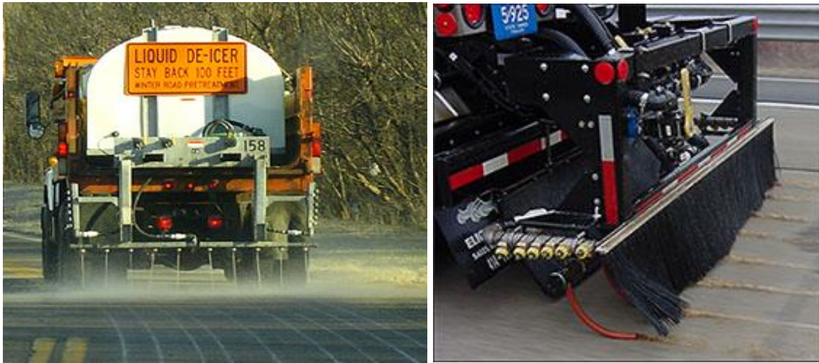
Figure 47: Anti-icing application to a road using stream nozzles
