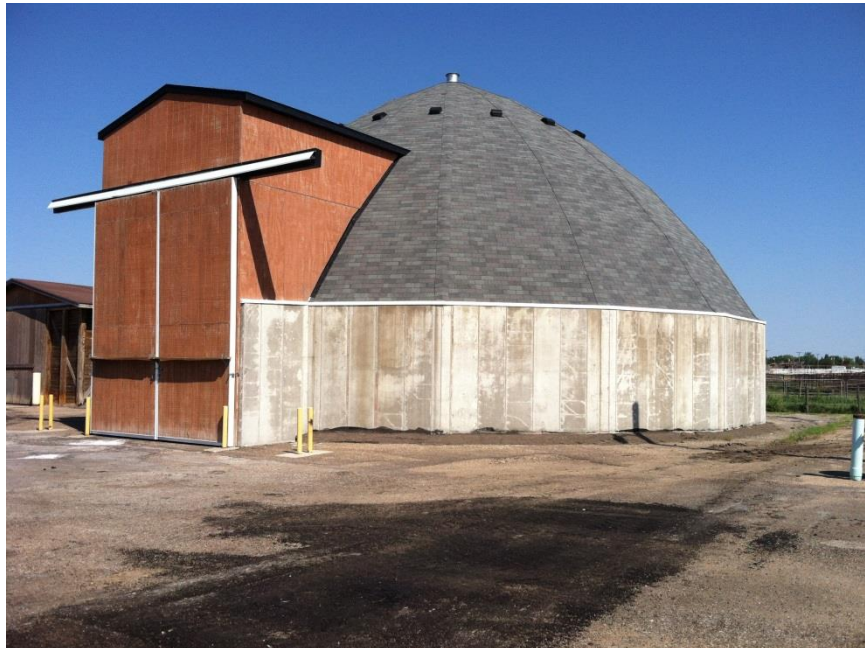
Figure 40: Salt dome style salt storage structure with a barn door and paved loading pad. Photo courtesy of Kansas DOT
