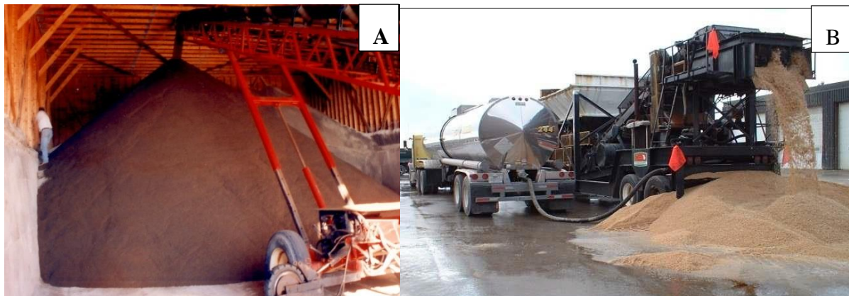
Figure 43: Pre-wetting, A) at the stockpile in storage and B) pre-wetting road salt prior to storage on impervious surface (Photo credits: Wilkinson Corp. and www.organicdeicing.com )
