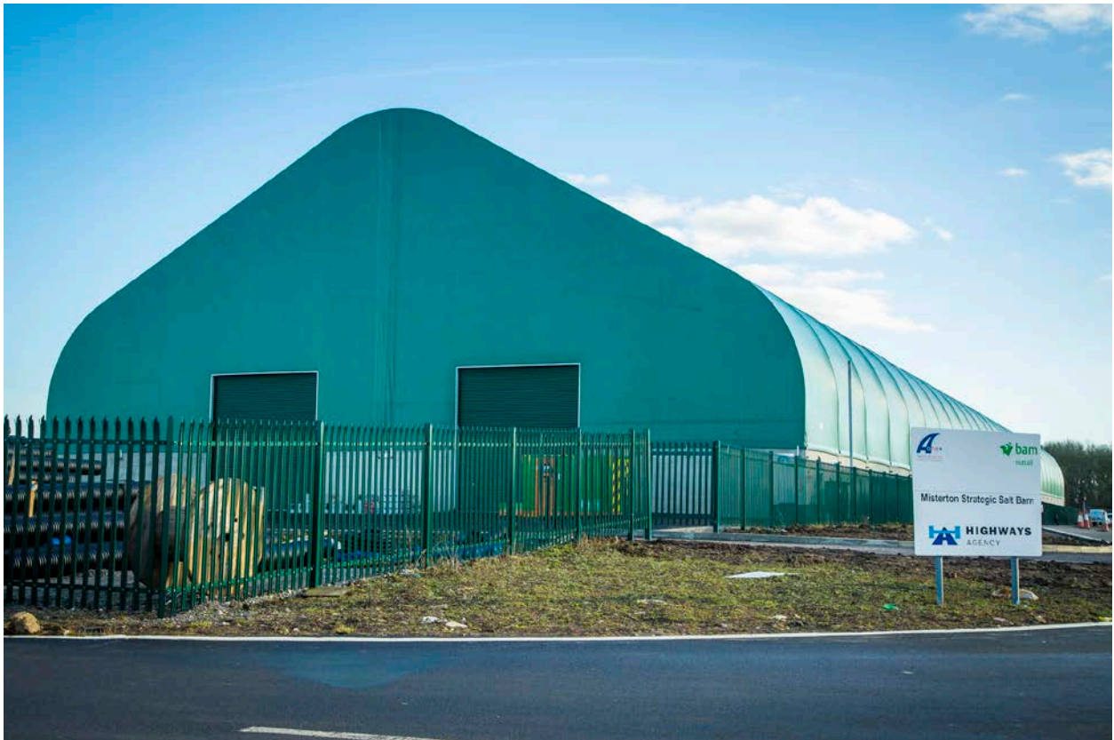
Figure 4-6 UK Salt Storage Facility
