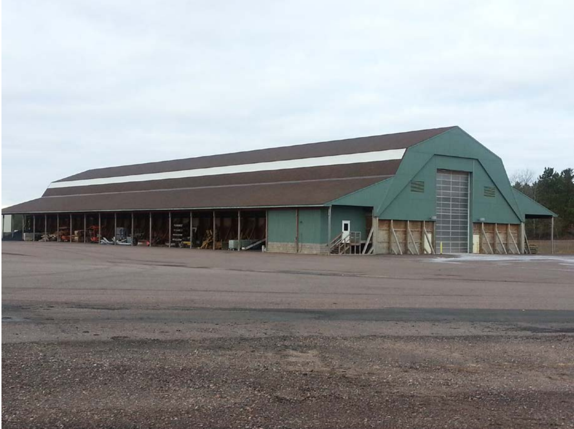
Figure 4-5 Additional Equipment Storage around Salt Barn
