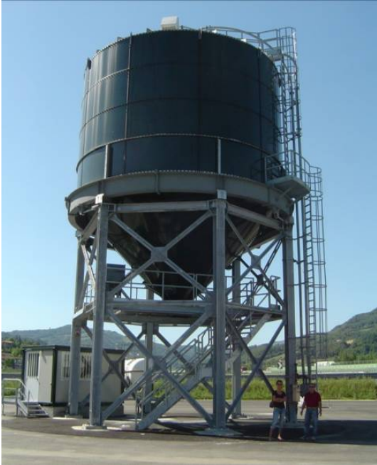
Figure 4-4 Silo Loading System from Europe
