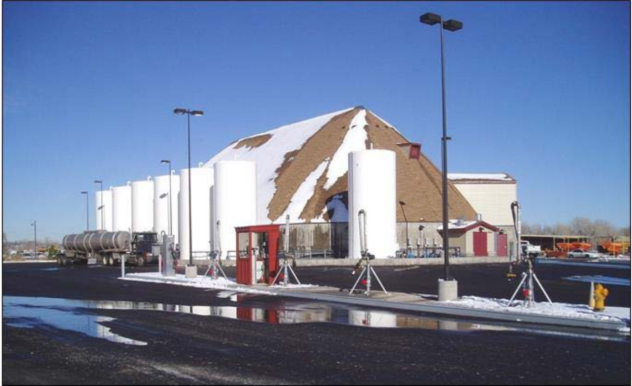
Figure 4-2 Salt Storage Facility Showing Multiple Access Points for Different Materials
