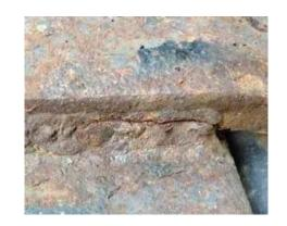
Rust jacking (a kind of corrosion fatigue) is the displacement of building elements due to the expansion of corrosion products.
