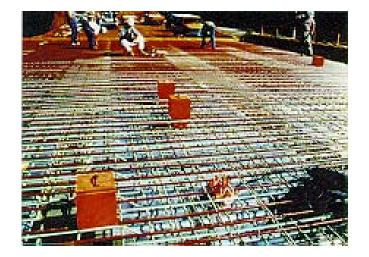
Figure 2.7 Deck heating system in the Buffalo River Bridge, Amherst, Virginia, 1996
