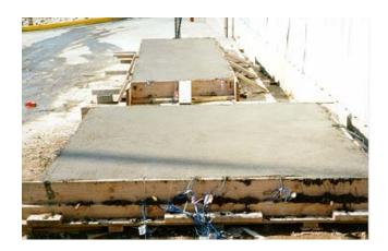
Figure 5-6 Slabs after finishing
