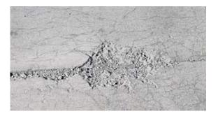
Figure 2.1 D-line cracking spreading from sidewalk joint
