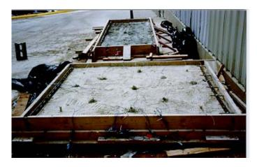
Figure 5-9(b) Thermocouple layout before casting overlay
