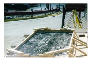
Figure 5-1(b) 6-in. conventional concrete layer
