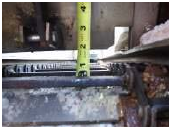
Figure 6-2 Selection of an appropriate single gate opening for range of application rates to be used.
