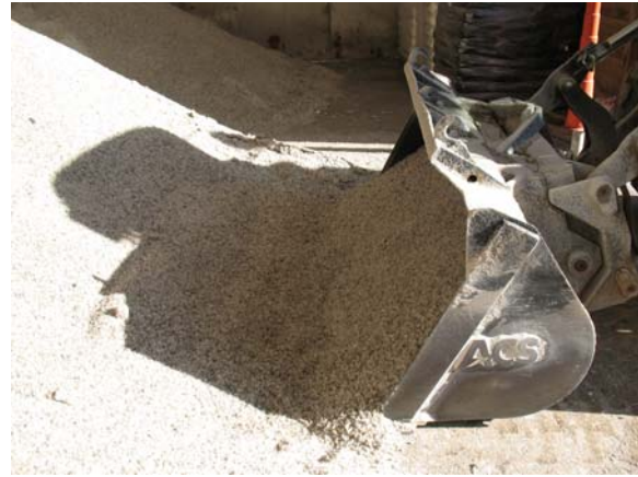
Figure 4-5 Mechanized loader bucket used to load spreader truck.
